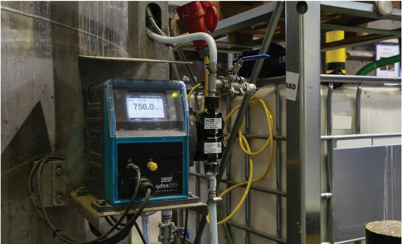
Above: A Qdos 120 pump used for dosing lime slurry
