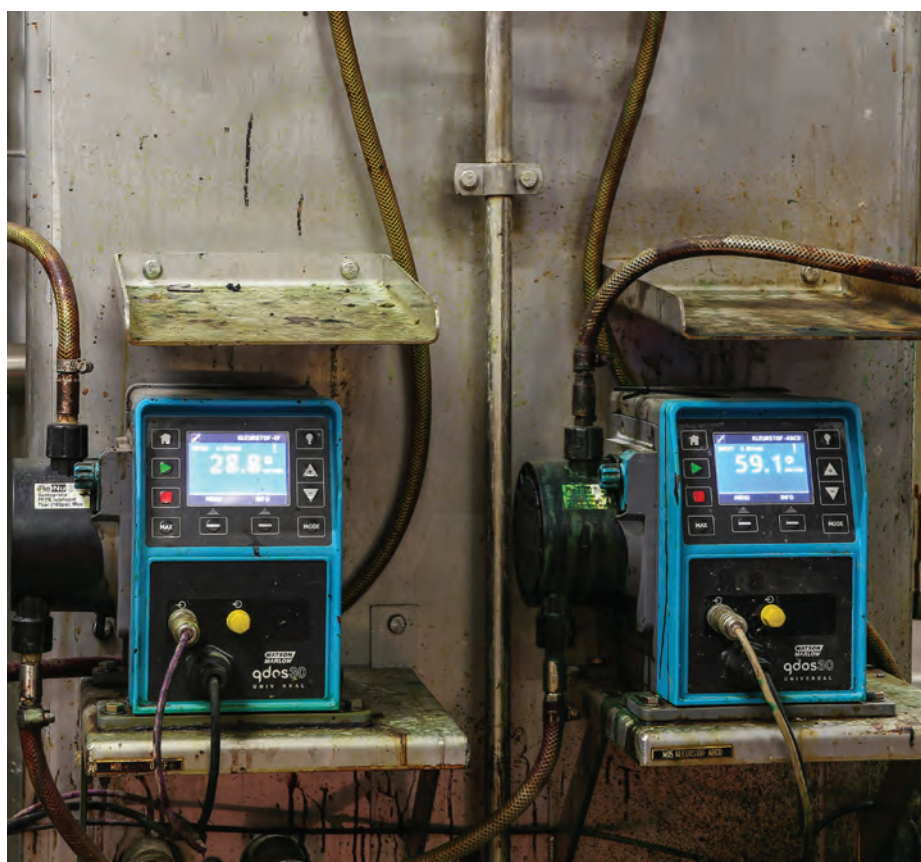
Above: Qdos pumps used for colourant dosing
