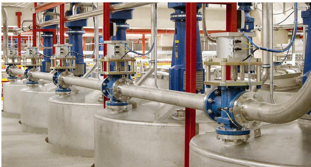
Picture 2 – Pigging line with distribution valves serving storage tanks
